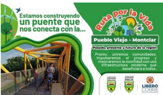
Figure 7 – New Montclar walking bridge under construction. (CNW Group/Libero Copper & Gold Corporation)
