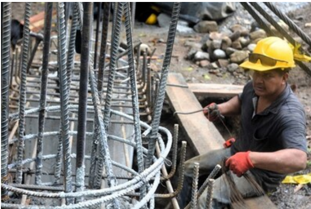
Figure 7 – New Montclar walking bridge under construction. (CNW Group/Libero Copper & Gold Corporation)
