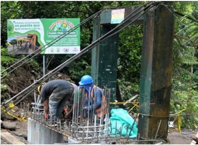
Figure 7 – New Montclar walking bridge under construction. (CNW Group/Libero Copper & Gold Corporation)
