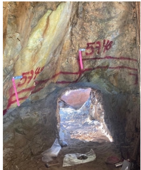
Figure 10 Left: Mineralised structure in the Copalquin Creek important for the overall district geologic model. Right: Inside the historic Copalquin mine showing diamond saw channel sample.
